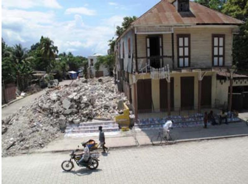
**A concrete structure (left) and a wood structure (right). Everyone in the house on the left perished when the earthquake hit. The building on the right is centuries old. It survived the earthquake and the many hurricanes throughout the years and sustained only minor damage.**
